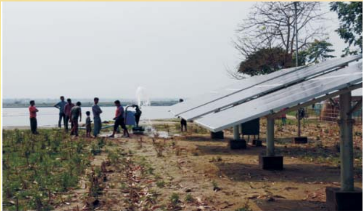
Solar Sprinkler Irrigation System under Enclave Development Programme at Karijabhatrigach, block- Dinhata-I, dist- Cooch Behar
