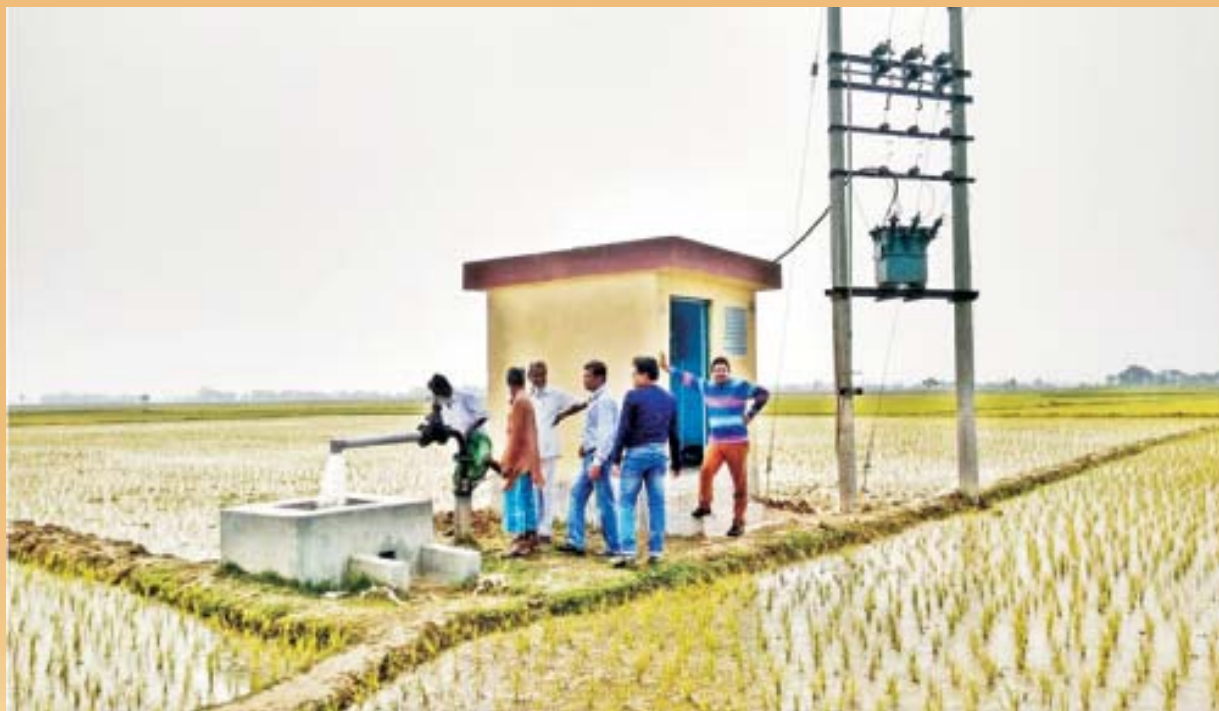
Operation of Tubewell scheme at mouza- Dasdebgram, dist- Murshidabad
